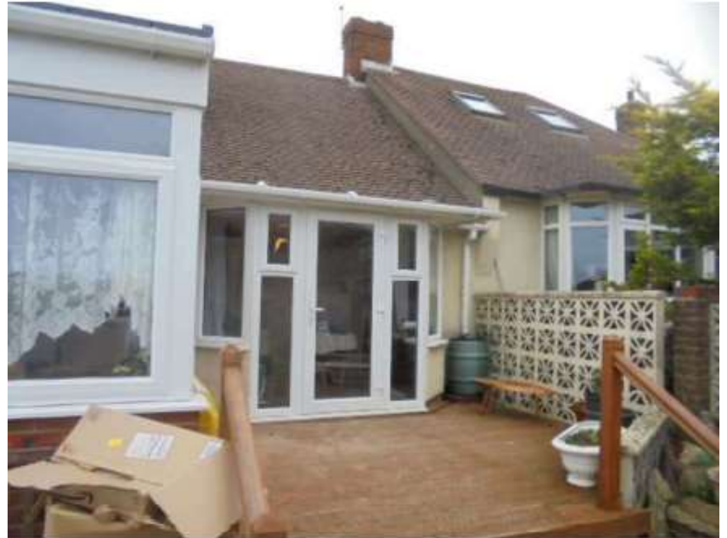
From rear – adjoining 120 Foredown Drive. Location of extension
