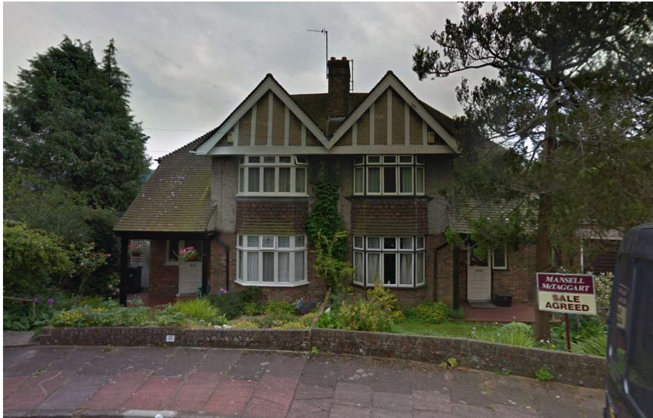
46 Ridgeside Avenue is on the right
